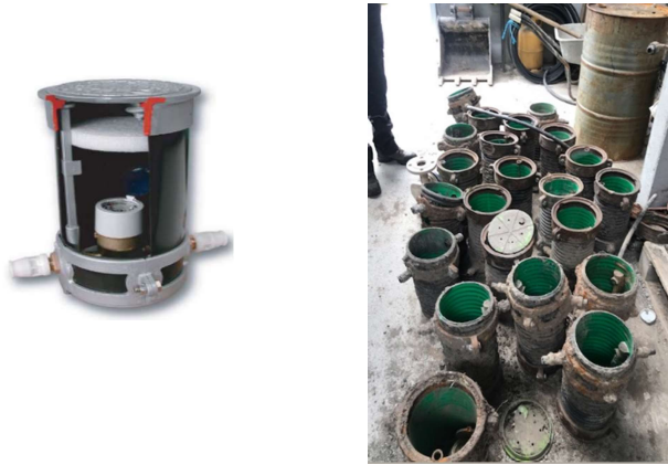
Figure 2: A WSC-R customer access box and some of the old WSC-R boxes after being replaced
